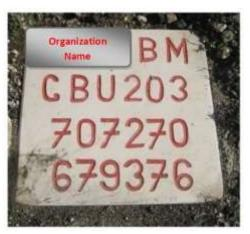
unsuitable for the terrain, then the LMAC may authorize an alternative fixed natural or manmade object for use as a benchmark. The same information as detailed above should be permanently recorded on the benchmark.
